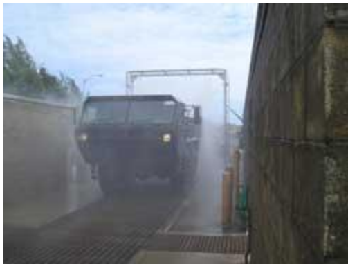
An LVS passes through one of two automated wash racks installed in 2005 at Marine Corps Base Kaneohe Bay on Oahu, Hawaii. Photo courtesy of the Marine Corps CPAC Office.
