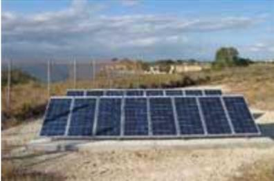
*Solar energy collected in this photovoltaic array provides power for a cathodic protection system that protects fuel and water pipelines at U.S. Naval Station Guantanamo Bay. Photo courtesy of Naval Facilities Engineering Command (NAVFAC).*
