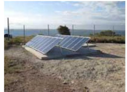
*The Navy has installed a solar-powered cathodic protection system on its base at Guantanamo Bay, Cuba. Photo courtesy of Naval Facilities Engineering Command (NAVFAC).*
