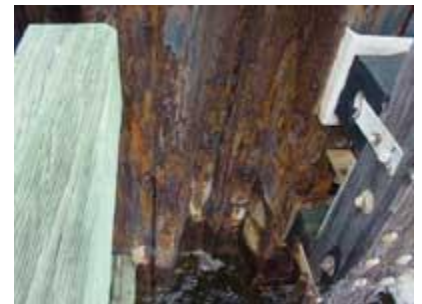
Pictured (top) is typical corrosion on steel piling at Naval Air Station Pensacola. A technician (bottom) applies a high-performance coating to the piling in order to protect the splash zone.
