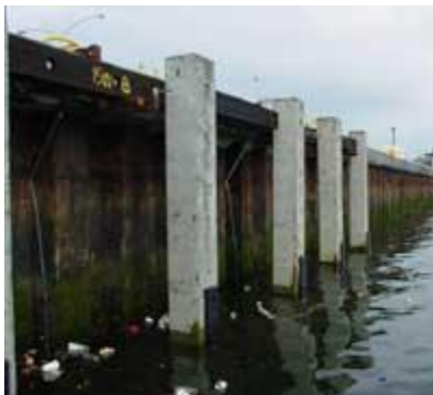
Sea water immersion and splash, pollution, and ultraviolet light exposure corrode the steel and concrete bulkheads at Naval Air Station in Pensacola (above), and the Naval Station on the eastern shore of San Diego Bay (below). Photos courtesy of Naval Facilities Engineering Command (NAVFAC).
