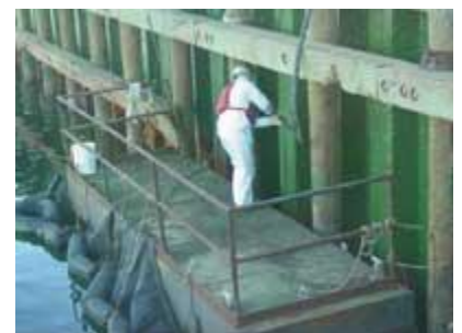
Pictured (top) is typical corrosion on steel piling at Naval Air Station Pensacola. A technician (bottom) applies a high-performance coating to the piling in order to protect the splash zone.
