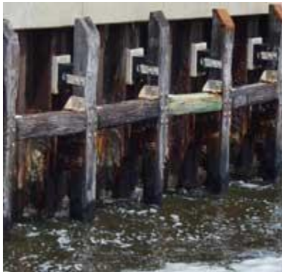
Sea water immersion and splash, pollution, and ultraviolet light exposure corrode the steel and concrete bulkheads at Naval Air Station in Pensacola (above), and the Naval Station on the eastern shore of San Diego Bay (below). Photos courtesy of Naval Facilities Engineering Command (NAVFAC).
