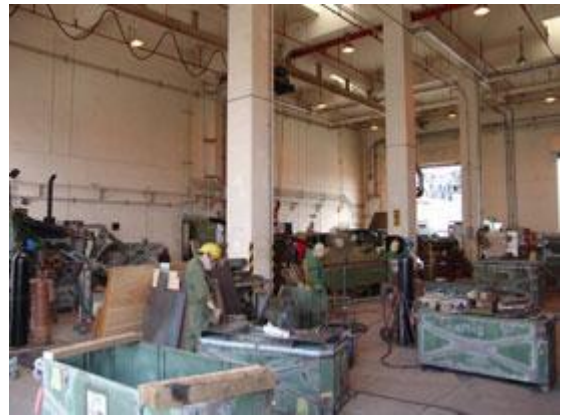
During 2012, the corrosion evaluation team will visit sites similar to this corrosion rehabilitation facility at Camp Kinser, Okinawa. The facility includes four double bays for performing vehicle body work. Photo courtesy of Marine Corps Corrosion Prevention and Control Program.
